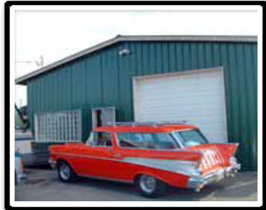
Exterior of Building
